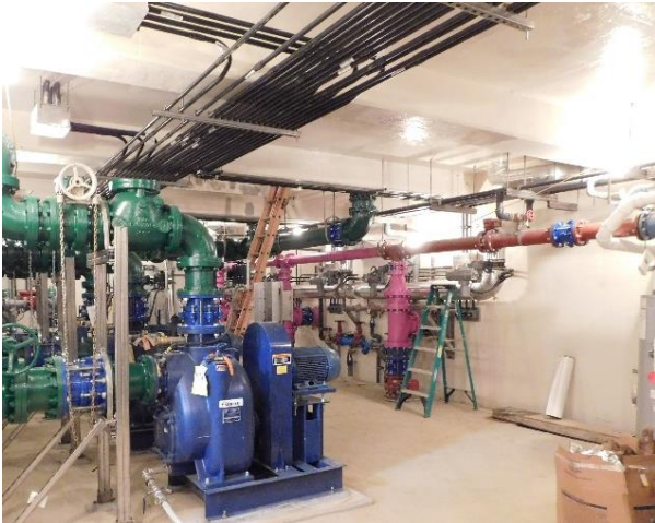
LEONARDTOWN WWTP PVC COATED RIGID
