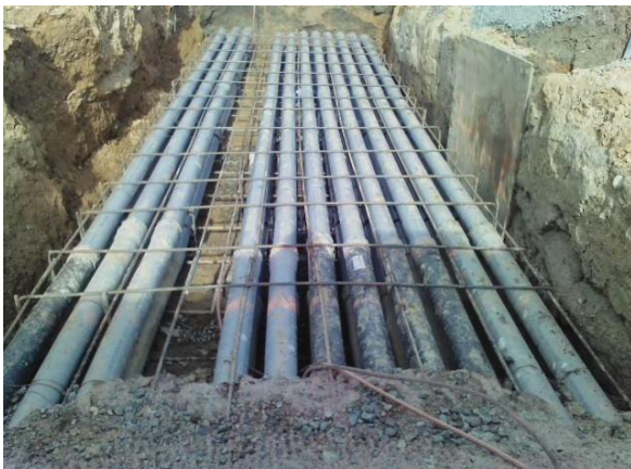
LEONARDTOWN WWTP DUCT BANK
